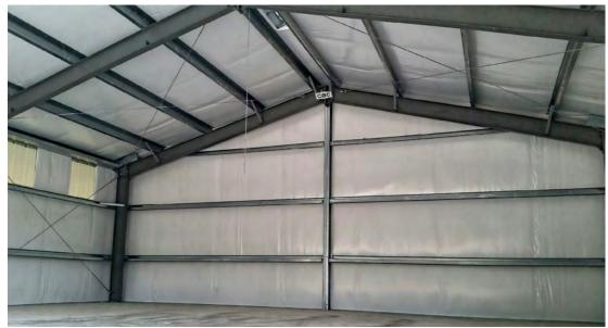
This storage building is a s  $40' \times 30' \times 11'$  custom built agricultural building made for storage of recreational vehicles and personal belongings. Fully insulated. Walls and doors with a 3' roof overhang at perimeter with R-panel soffit. Soffited overhangs all around with 4 wall lights per side for natural lighting.
