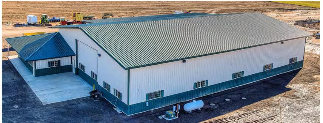
The Yeates Family Farm Shop is a 80' x 125' x 20.33' building with an added wood framed office and pump house that is clad in our Standard R Panel. This project has a 3' roof overhang at the perimeter with soffit, including a 23' x 100' x 19.83' Lean-to with 3' extension with an R-panel ceiling liner. One end has a 30' x 18'6" door and the other side has a 26' x 18'6" Hi Power door, and (2) 22' x 14' custom green sectional doors with a total of .
