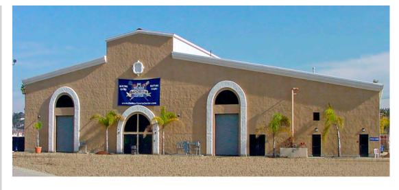
This sports facility was designed using a custom CBC building at 119' wide x 312' long clear span with a 29' x 4" eave and a 2:12 roof slope. A 31'-5" full length clerestory by 6'-8" high and a 38' x 98' lean-to. The roof panels are Standard R-Panels in Terra Cotta. All the walls are studs with stucco and masonry.
