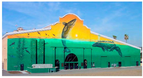
The Del Mar Wyland Event Center is a custom CBC building consisting of a 158' wide x 216' long clear span structure with a 36' eave height and a 2:12 roof slope. A 31'-5" full length clerestory by 6'-8" high and a 16' x 24' lean-to. The roof panels are Standard R-Panels in Terra Cotta. All the walls are studs with stucco and masonry. The north endwall features a painting by renowned marine life artist, Wyland to celebrate ocean conservation.
