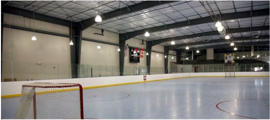
This 20,680 square-foot steel building is an indoor roller hockey arena. The main structure consists of a 94' wide x 220' long x 24' eave height structure. The roof is covered with our Standard R-Panel and features a stucco exterior finish.
