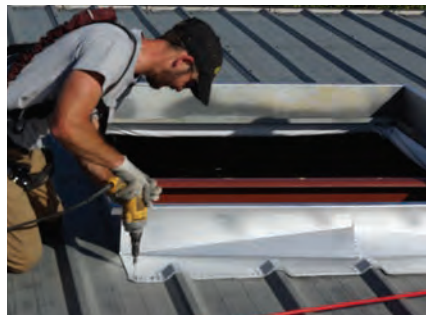
3. Install roof curb.
