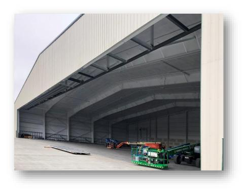
The first hangar, with completion coming by the end of August, is a 230' x 135' x 37' symmetrical gable building with a 24' x 120' x12' low-eave lean-to. The lean-to is located off the left end wall and will be finished as office space.
